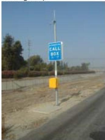
"B" site is on an upward slope and is "in cut" into the slope/hill. Most often requires transverse walls.
